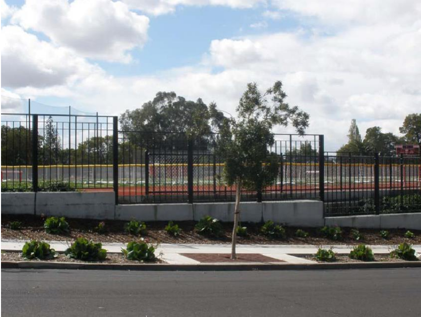
Image 44 – St. Mary's street walls along Posen Avenues
