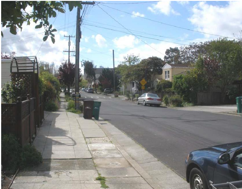
Image 20 –typical southern Neighborhood Street, looking into Berkeley
