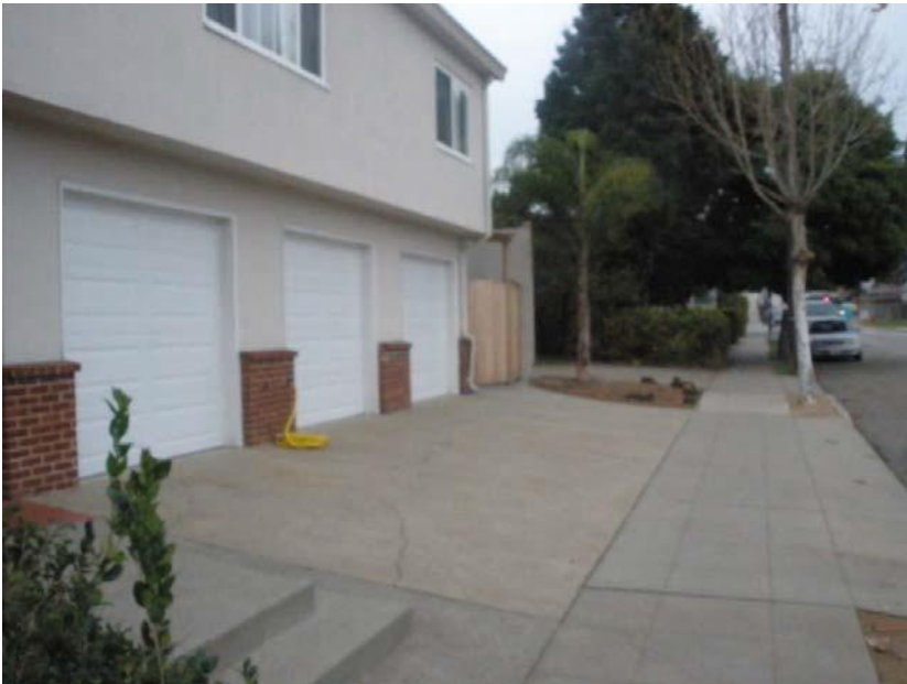
Image 33 –Apartment garages – doors/ façade opportunity here
