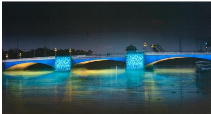
Tracey Dear, Agua Luces Kennedy Boulevard Bridge - Tampa, FL
