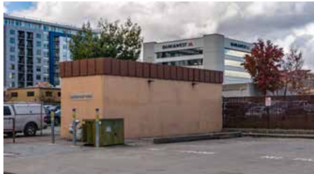
Water pump stations
