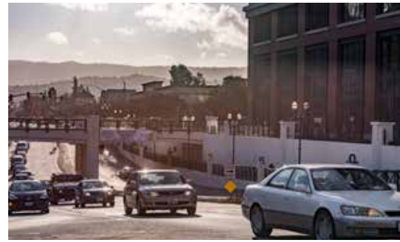
Jefferson street underpass wall
