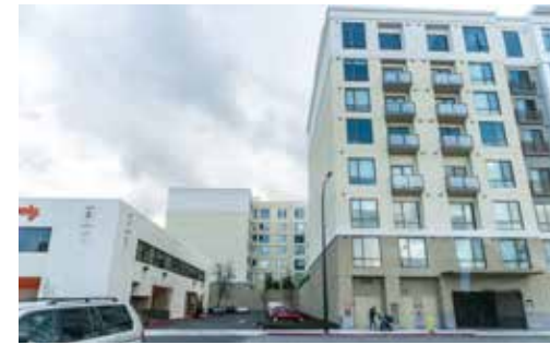
marston by Windsor walls
