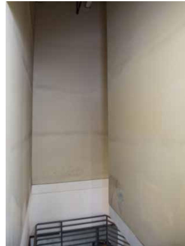
Jefferson Garage stairwells
